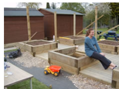
Fit deck and place gravel
